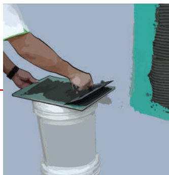
8. Apply grout (Creteplus-TE + Cement + Water) to the tile
