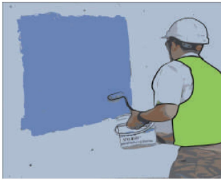
1. A layer of BA666 on substrate. Wait until surface dry estimate 30 minutes - 1hour (Depending on weather condition)
