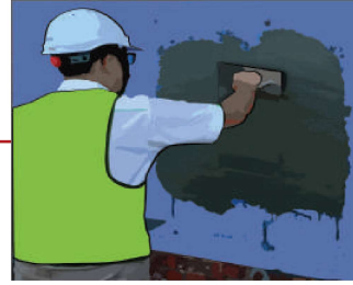
6. Proceed with plastering on treated substrate
