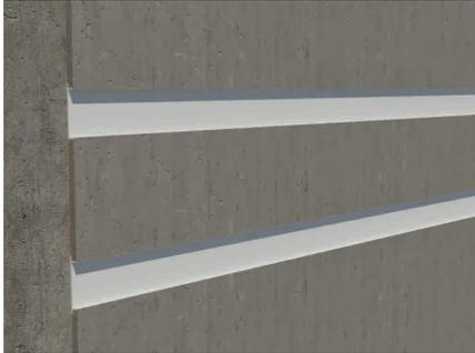
2. It is used as a throating line to prevent the rain water backflow and eliminate water marks/stain at external wall, internal wall and ceiling.
